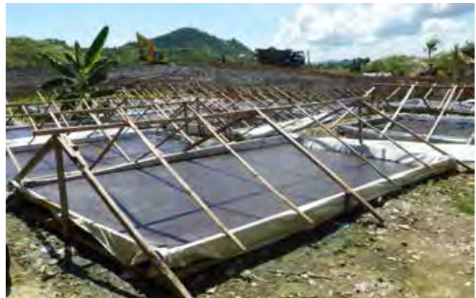
Figures 10 and 11. Sand drying beds (left) showing characteristic “cracks” on the sludge surface, indicating sludge is sufficiently dewatered to transfer to bulk biosolids storage area (about 25% dry solids). Sludge drying beds (right) with canvas tents (removed) to shed stormwater which allows dewatering even during rainy season.
