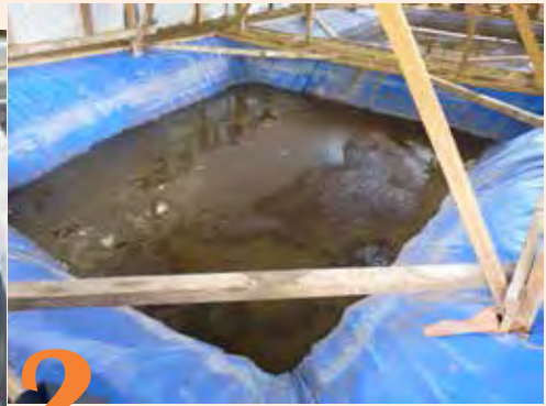
Reactor tank where lime and septage are mixed
