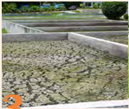
Sand drying beds with underdrains
