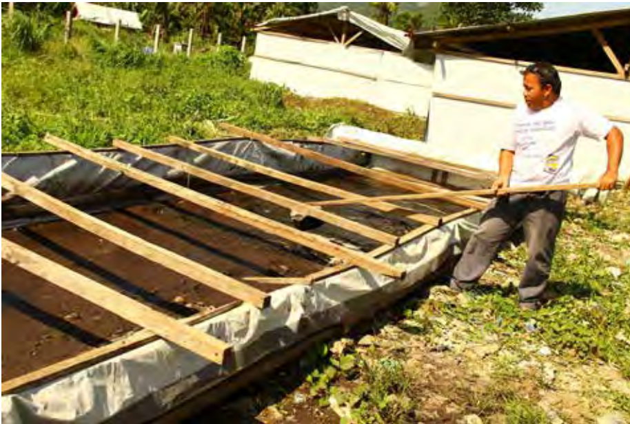
Figure 27. Worker levels stabilized sludge in a makeshift drying bed in an effort to keep biosolids on site in Tacloban City.
