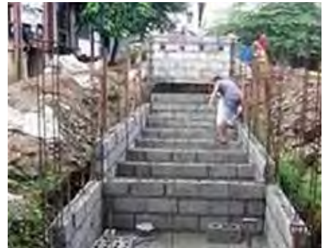
Figure 14. Anaerobic baffled reactor under construction.
