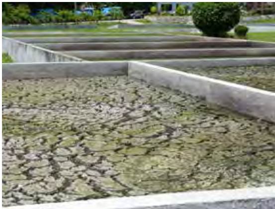
Figures 10 and 11. Sand drying beds (left) showing characteristic “cracks” on the sludge surface, indicating sludge is sufficiently dewatered to transfer to bulk biosolids storage area (about 25% dry solids). Sludge drying beds (right) with canvas tents (removed) to shed stormwater which allows dewatering even during rainy season.
