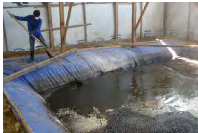
Figure 26. This is a reactor pit in Palo, Leyte, which was first built after Super Typhoon Yolanda. Here, workers stabilize the septage with lime, then transfer it to sand drying beds.
