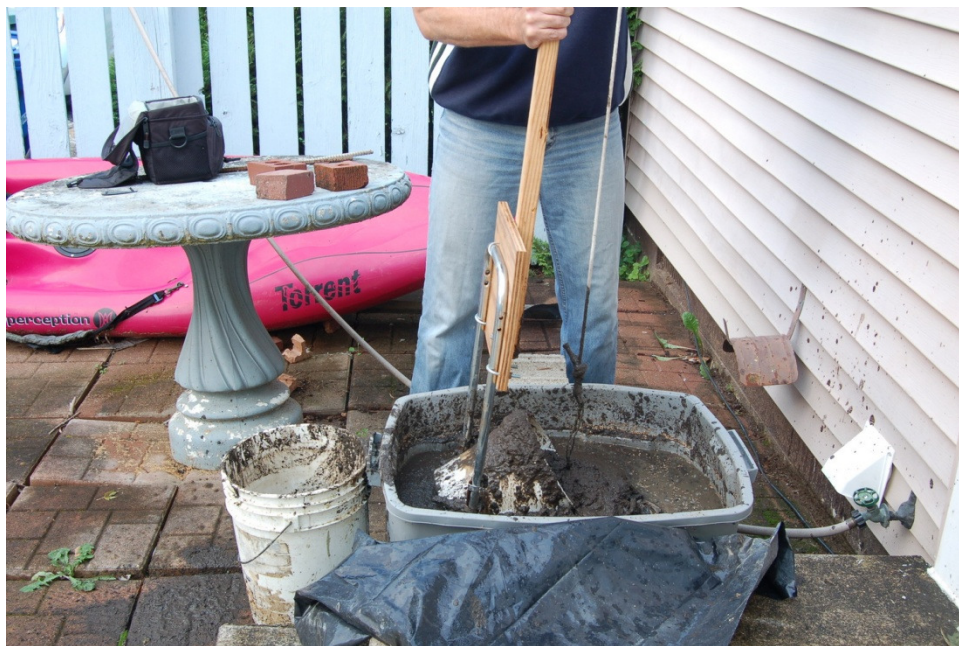
Figure 5: The rope is pulled up with the left hand while the handle is held in the right. The bucket rotates up. After this, the bucket is pulled up and dumped in the same way as with the thinner material, shown in Fig. 3.
