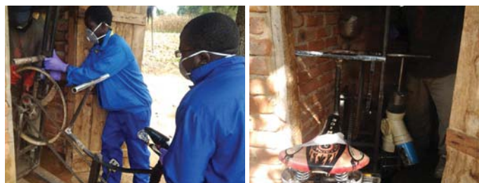
Figure 5: Modified pedal transmission mechanism being carried inside the pit latrine (a) and attached with the Gulper technology inserted in the sanitation keyhole (b).
