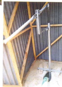
The suction hose pipe makes the pit emptying operation cleaner.
